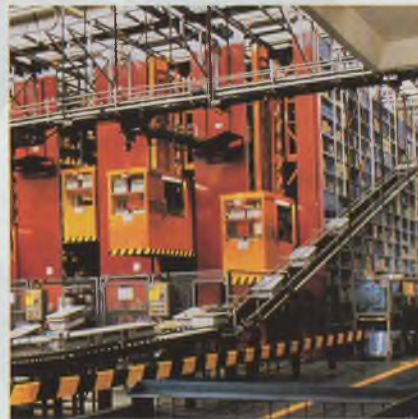
The central parts facility in Kassel, West Germany has automatic parts retrieval systems to expedite distribution.
